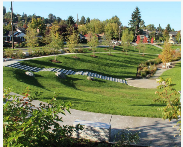
A stormwater park in Madison Valley helps manage drainage and beautifies the neighborhood. Photo: Seattle Public Utilities.
