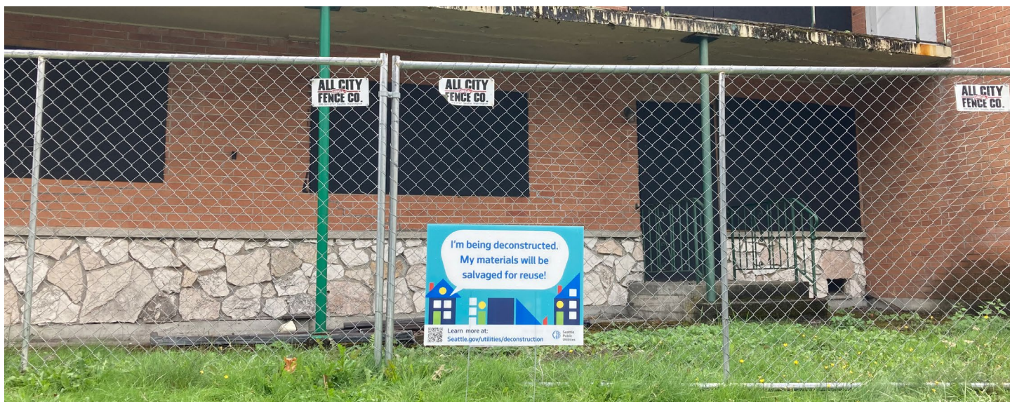
A building demolition site collecting salvaged materials for reuse. Photo: Seattle Public Utilities.
