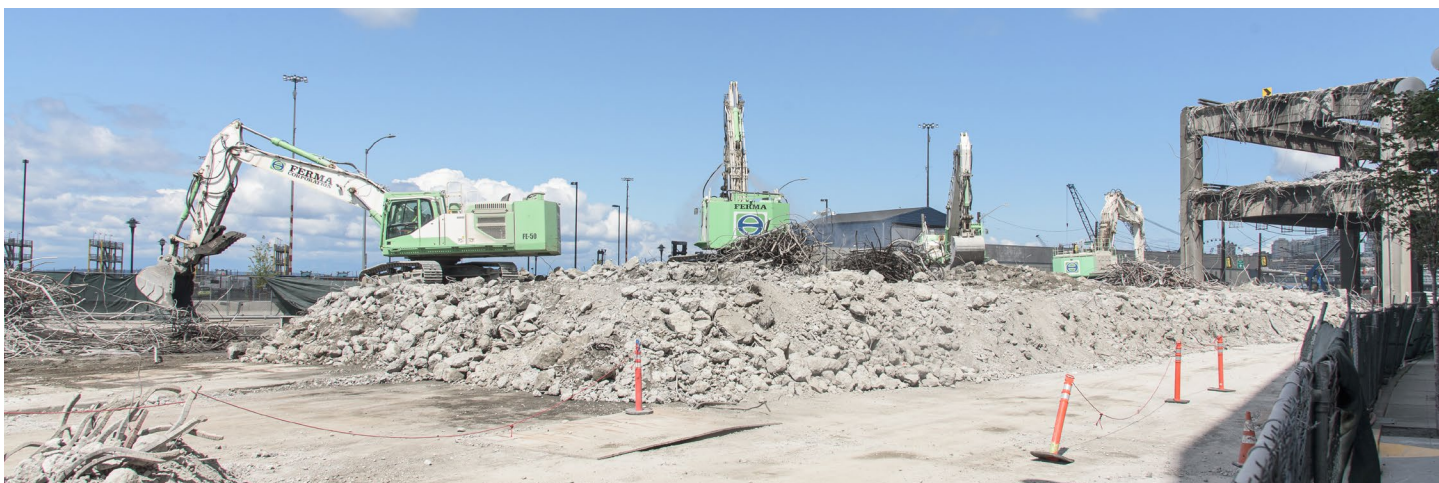
Sorting demolition rubble for recycling. WSDOT, Flickr Creative Commons .
